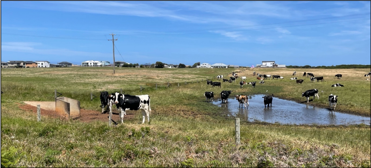
Figure 31 Southwest view of stormwater outfall
