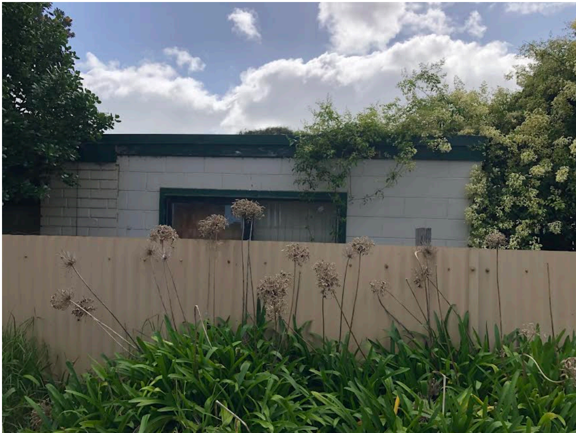
Figure 21: Example of construction on corner block in Port Fairy. Outbuilding associated with house on corner of Albert and Polding Streets, Port Fairy situated within 1m of Polding St boundary.
