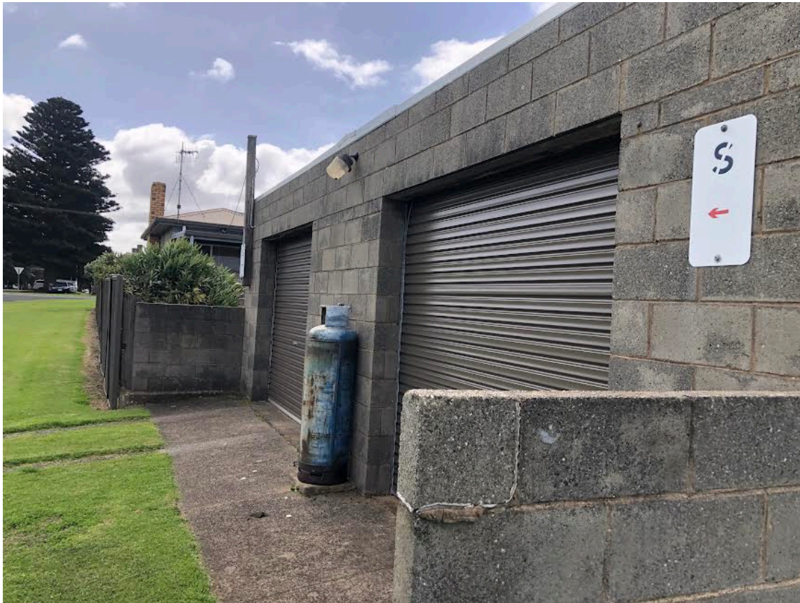
Figure 20: Example of construction on corner of Campbell and William Streets (70 Campbell St). Garage is within 1200mm of William St boundary.
