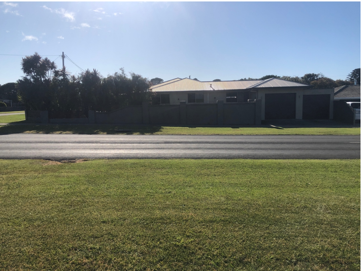
Figure 6: View of 12 Polding St from west (College St)
