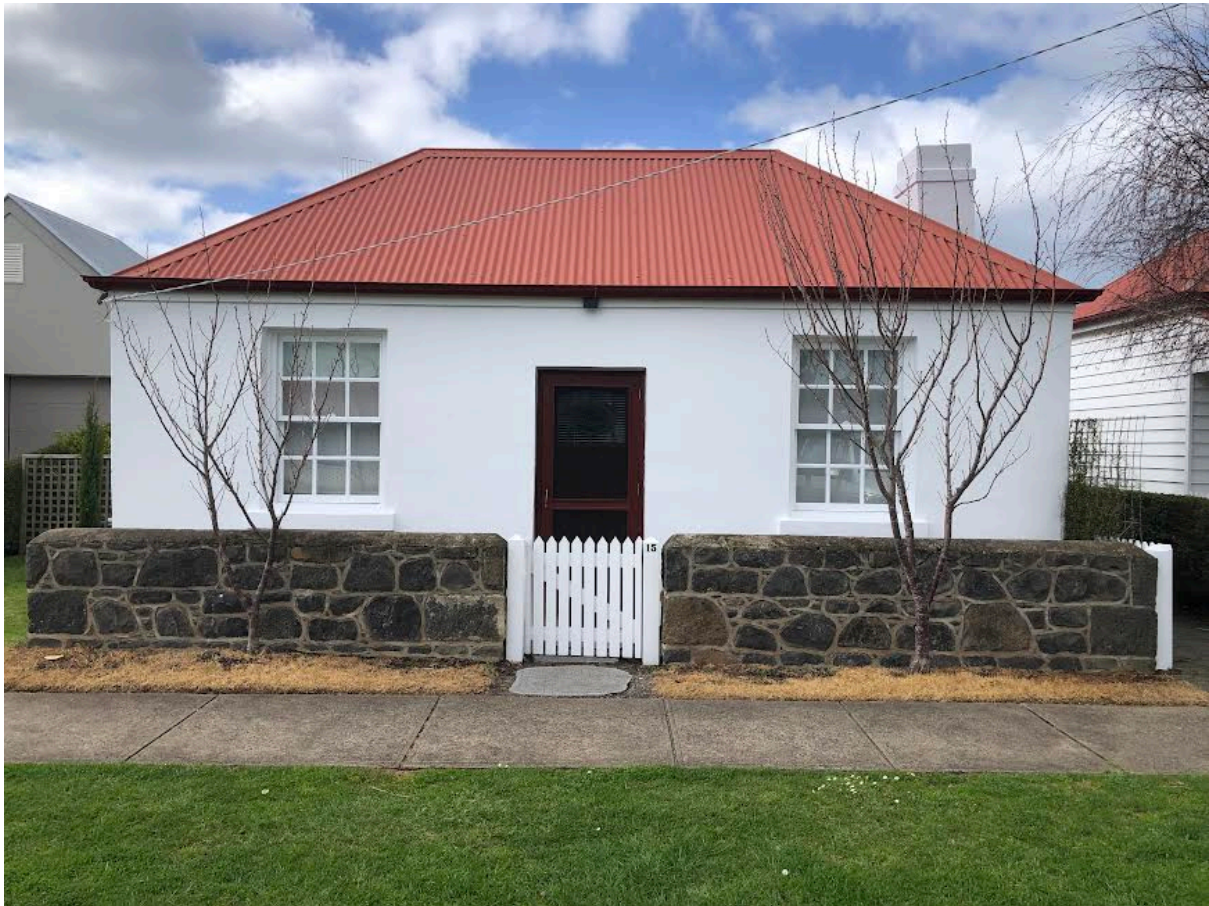
Figure 24 Example of construction close to property boundary with road. Whalers Cottage at 15 James St, Port Fairy located approximately 1m from front boundary.
