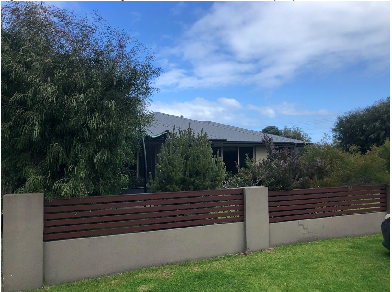
Figure 4: View of 12 Polding St From Northeast Corner of Property
