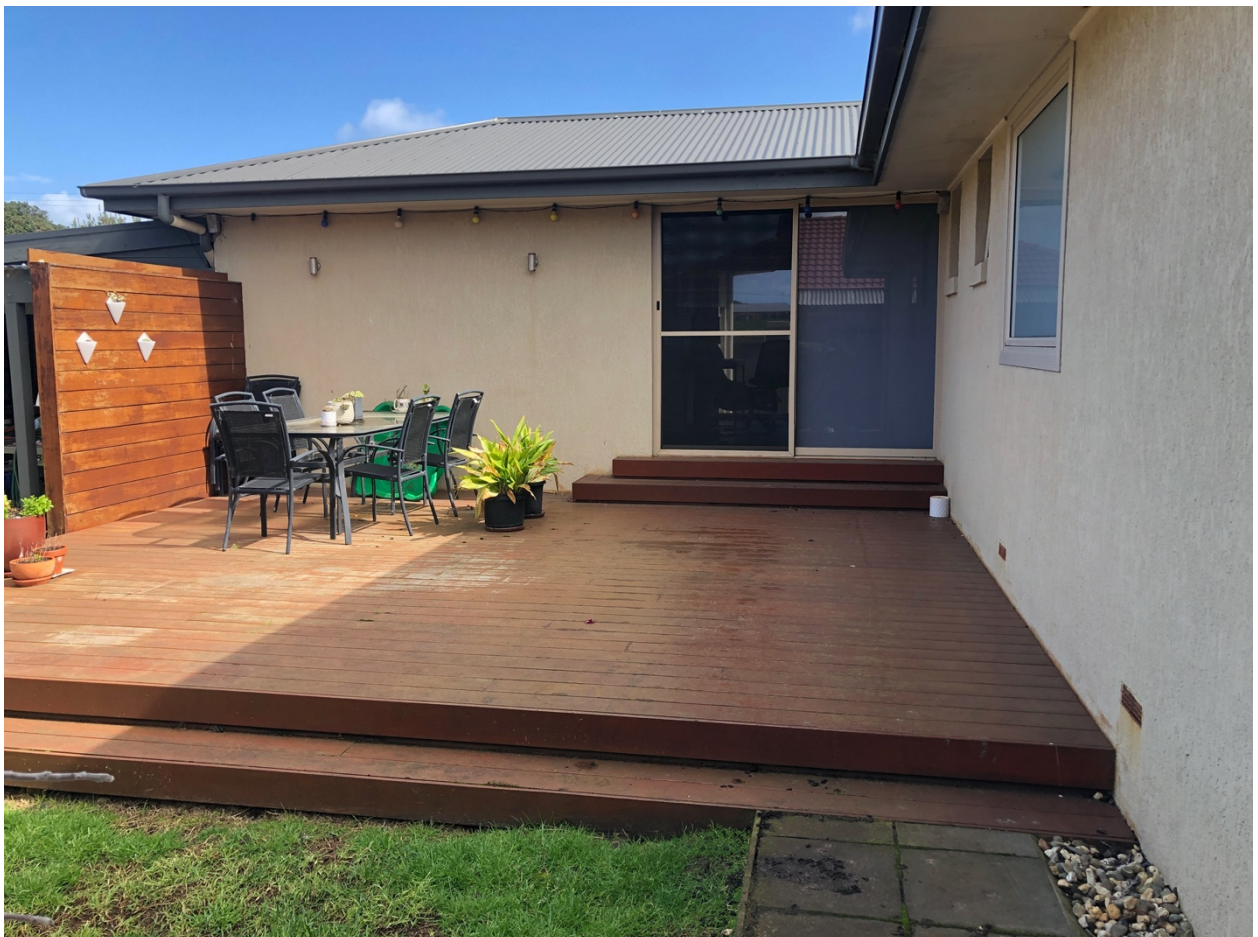
Figure 28 View of deck from east boundary.
