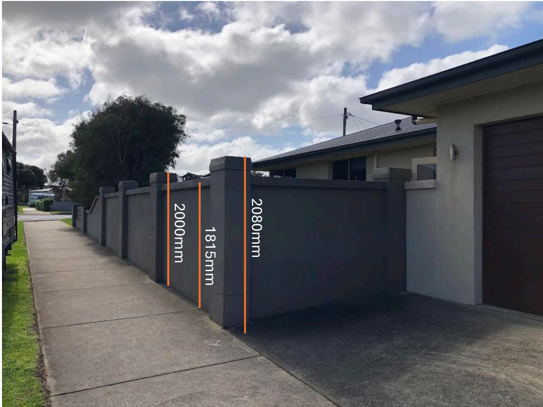
Figure 11: West facing boundary fence on College St. Midpoint on wall panel is approx. 1800mm and the two piers at either end of the panel approximately 2000mm.
