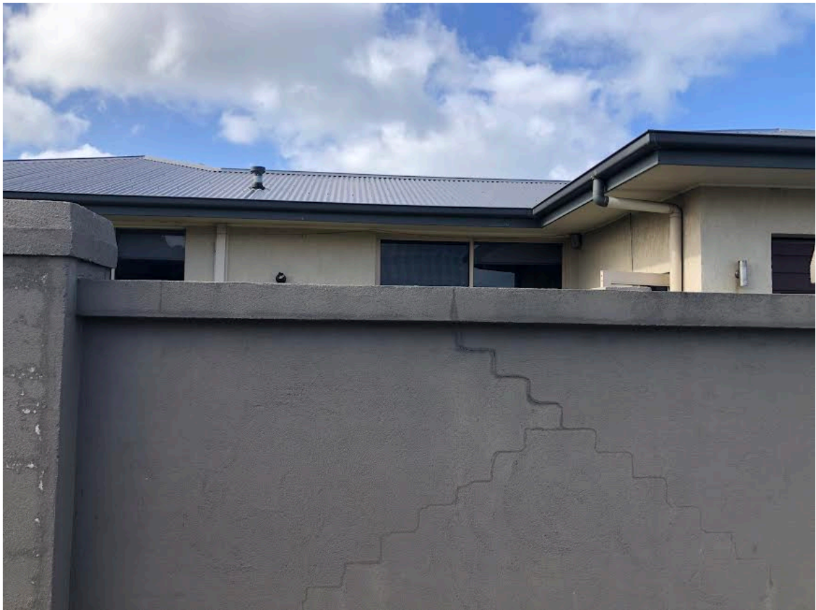
Figure 14: View of 12 Polding St from footpath on College St.
