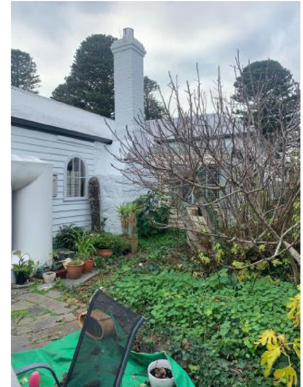
VIEW OF SOUTH WEST OF ORIGINAL BUILDING
