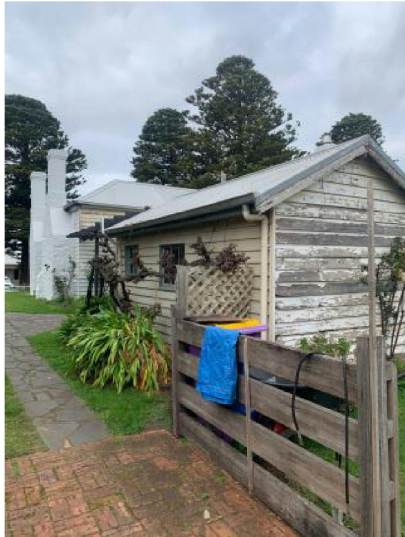
TRANPORTABLE ADDITION ON NORTH WEST
