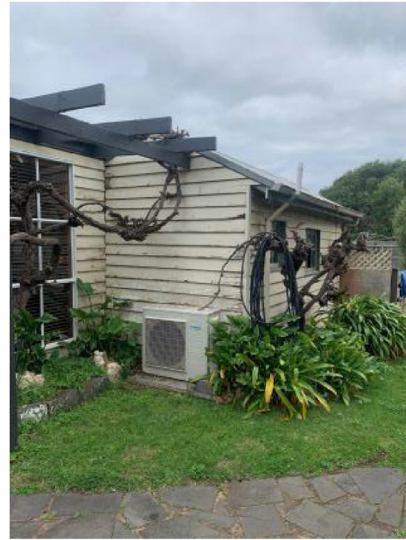
TRANPORTABLE ADDITION ON NORTH WEST
