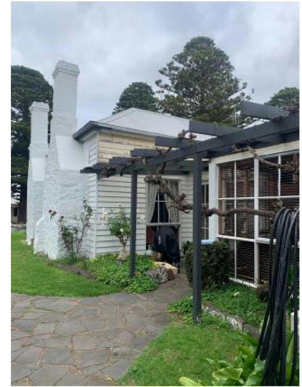
VIEW INTO NORTH WEST OF ORIGINAL COTTAGE
