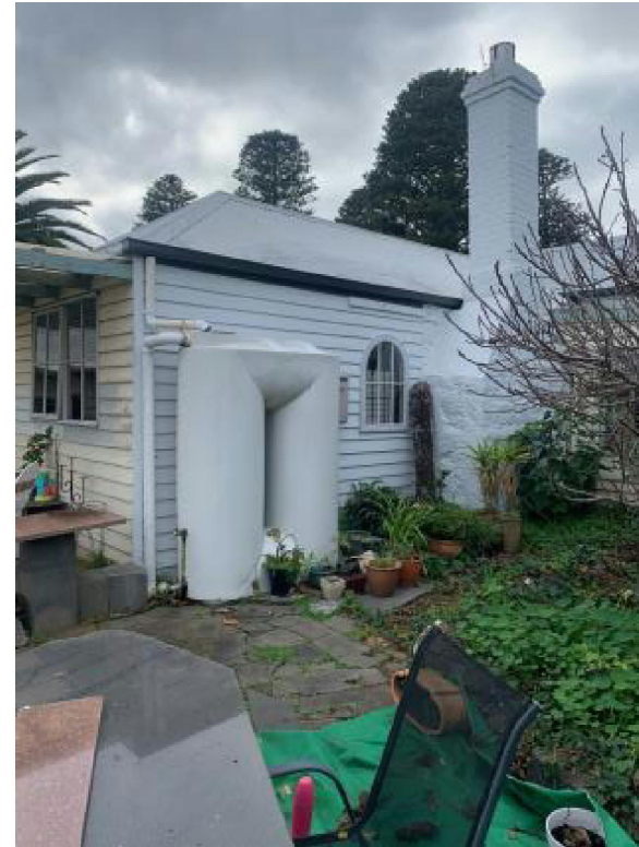
VIEW OF SOUTH WEST OF ORIGINAL BUILDING
