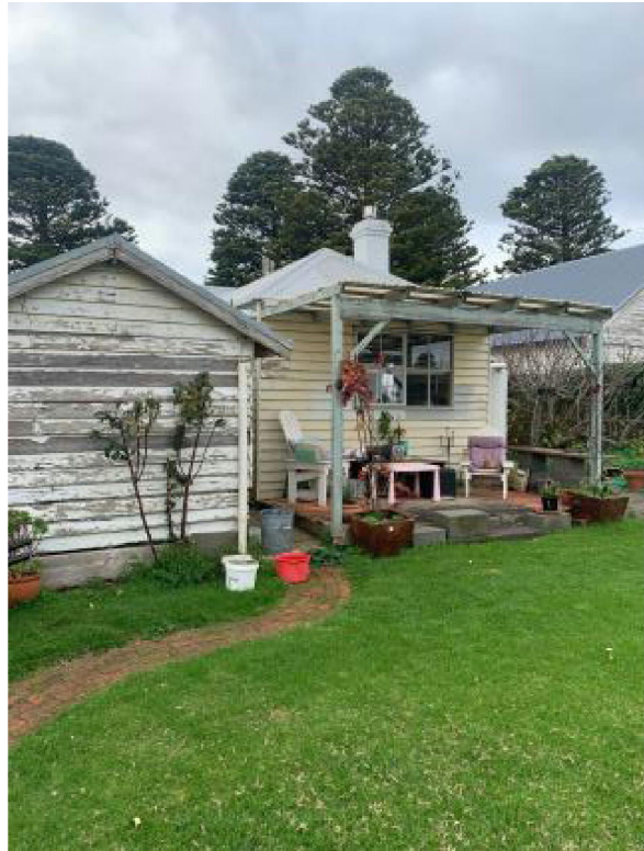
VIEW OF WESTERN FACADE (ORIGINAL BUILDING ON RIGHT)
