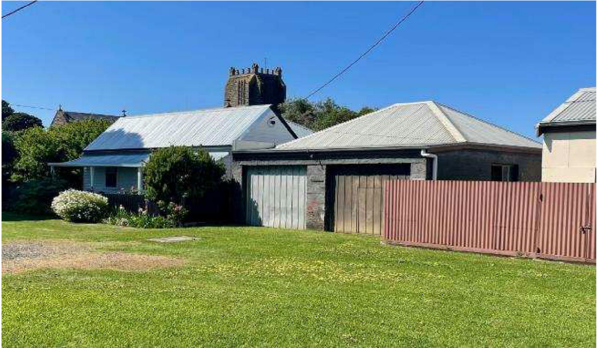
View from Regent Street of garages and abutting cottage
