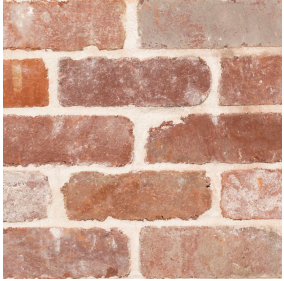
Feature wall at entrance: Recycled brick (as selected)
