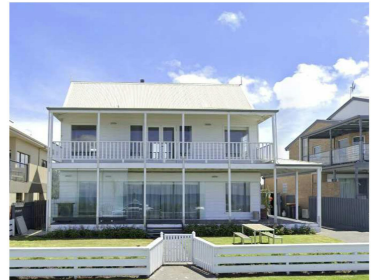
3 HANLEY COURT - DEMOLISHED
