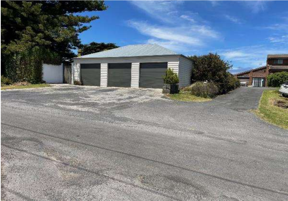
Garages of abutting property to the east
