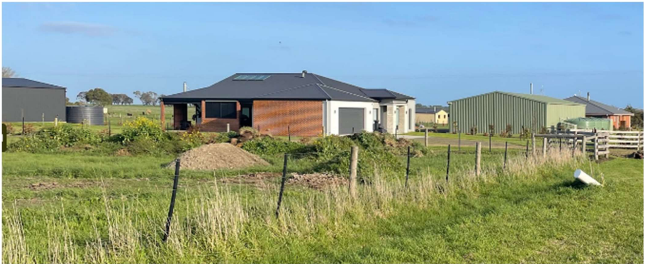
House under construction adjacent
