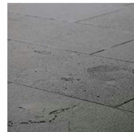
STN-02 TYPE: DIAMOND SAWN BLUESTONE TILE COLOUR: DARK GREY BLUE TONES EXTERNAL STONE PAVING & LANDSCAPE ELEMENTS
