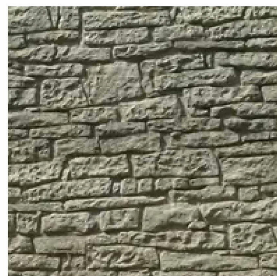
CON-01 TYPE: PRECAST CONCRETE WITH FORMED STONE TEXTURE COLOUR: SUBTLE EARTHY TONE MACHINERY SHED EXTERNAL WALLS
