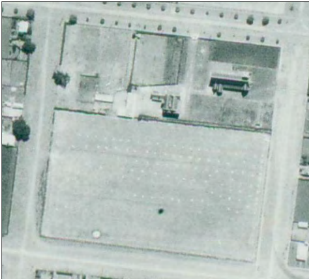
Figure 8 – The proposed development site in 1947 that includes the existing church building (Source: Trove 2024).
