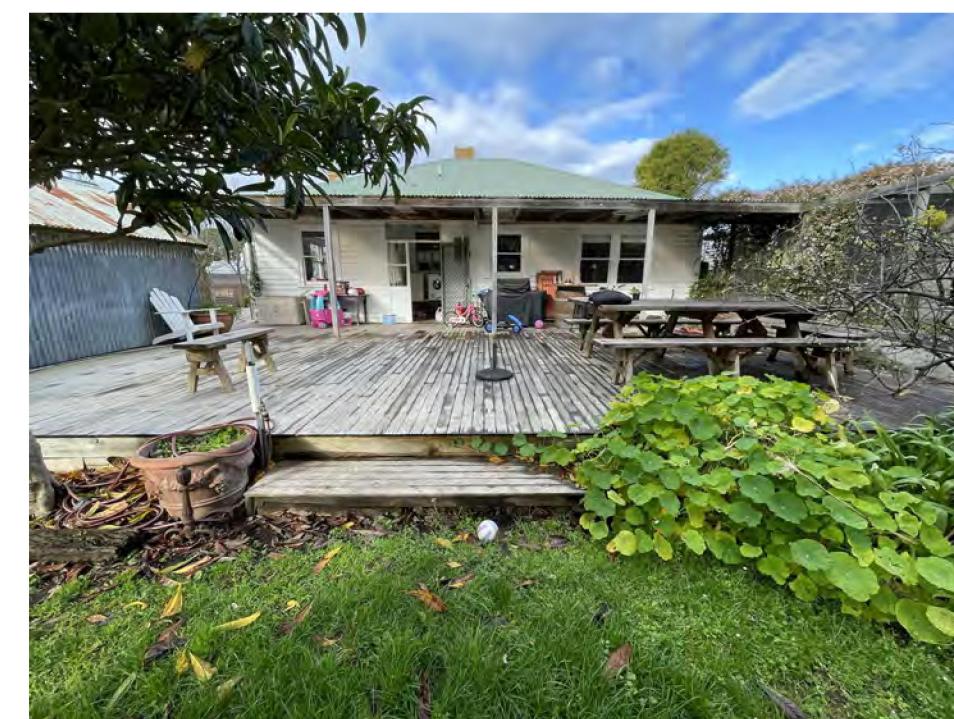
north facade of existing dwelling on subject site
