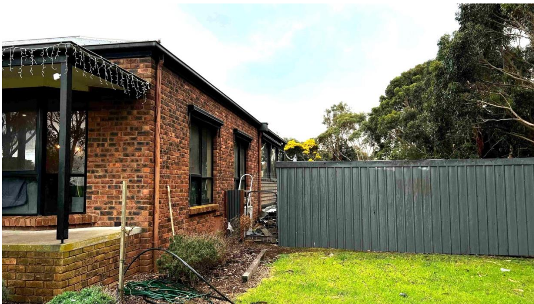
AREA OF ADDITIONS FROM FRONT (WOOD SHED TO BE REMOVED)
