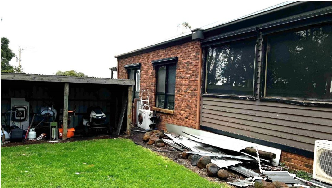
AREA OF ADDITIONS FROM REAR (WOOD SHED TO BE REMOVED)
