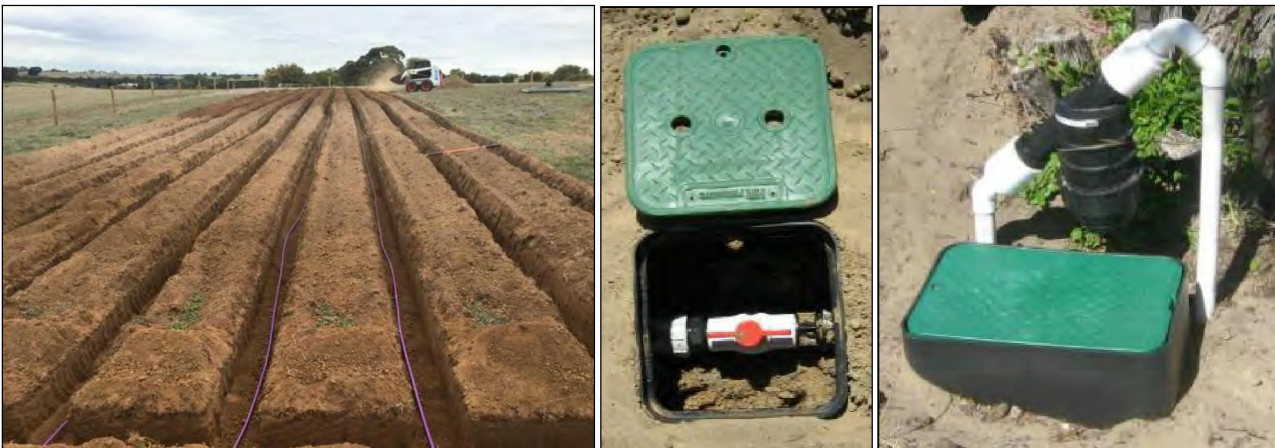
Figures 39-41 – Subsurface irrigation ground preparation; in-line valve, in-line filter.
