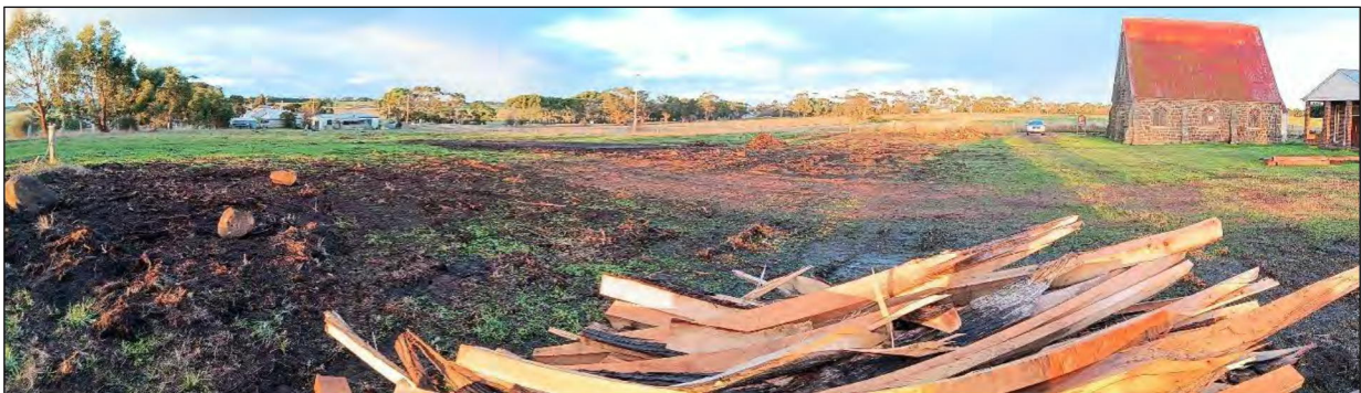
Figure 3 – Recent site clearing works have removed shading aged conifer trees to enhance potential wastewater disposal.
