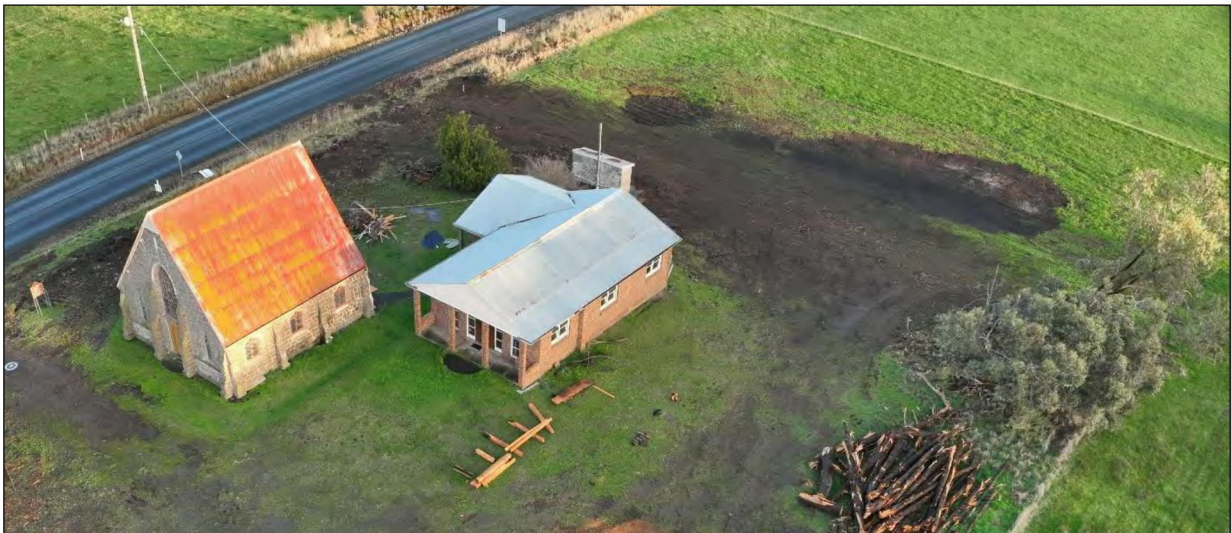
Figure 38 – Perspective view to the south-west over the existing church, hall, and adjacent areas for disposal.
