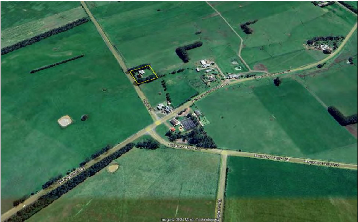
Figure 5 – The site exists within the northern part of the Russells Creek catchment (Source: Airbus 2024).
