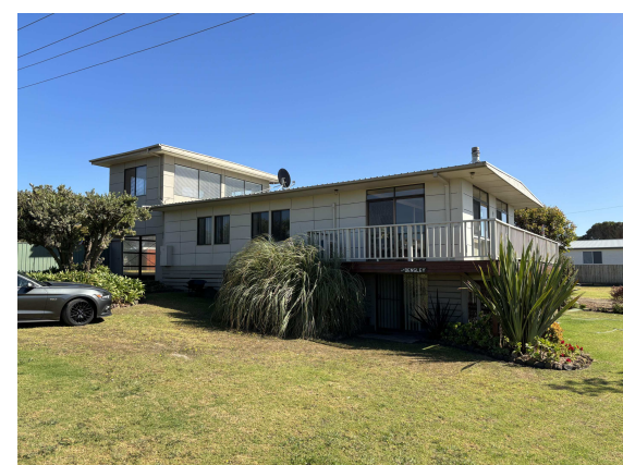
EXISTING SOUTH VIEW
