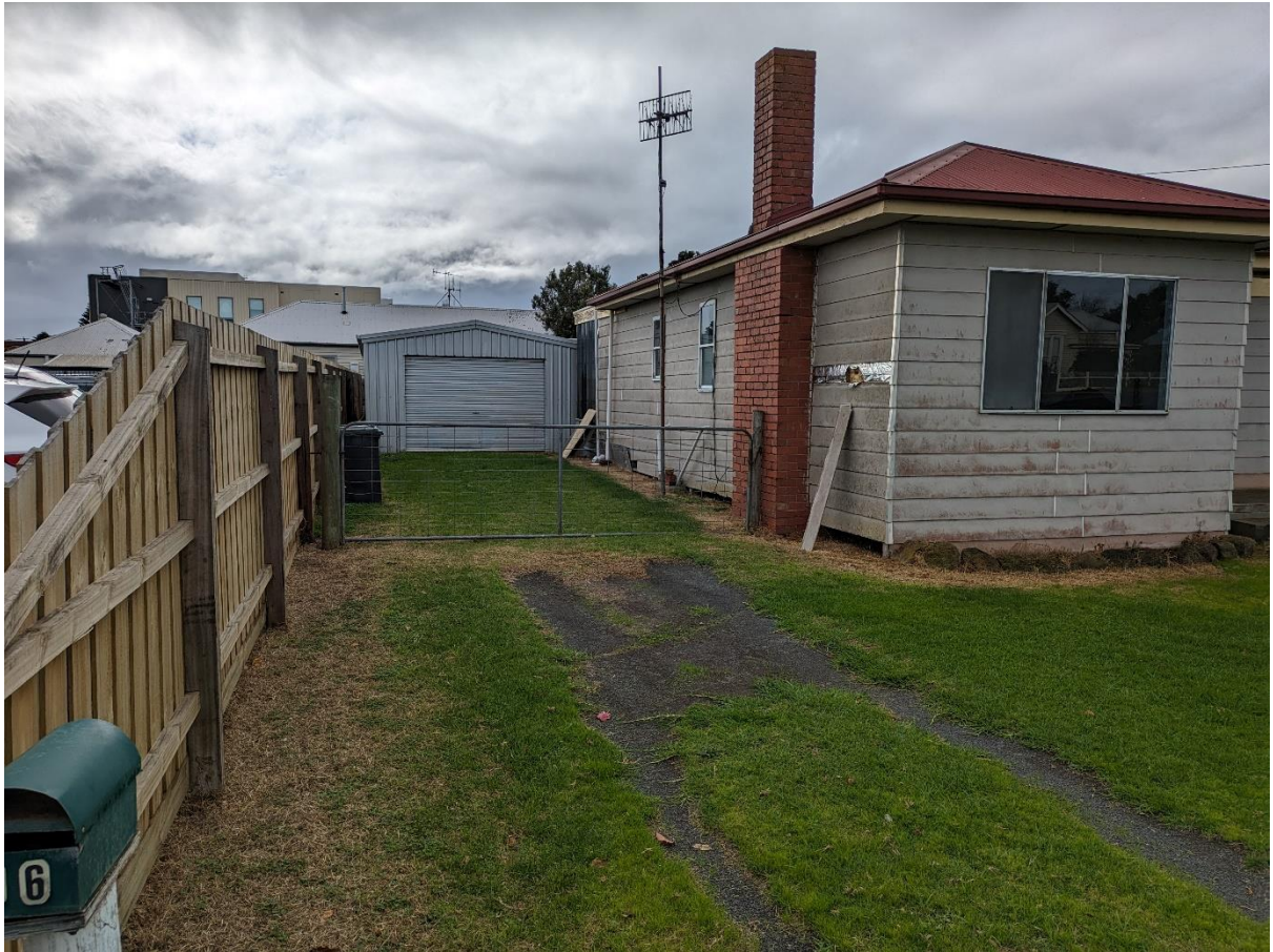
96 Bank St demolition
