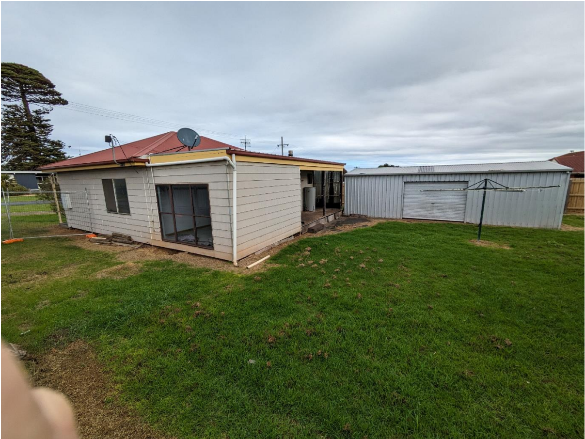
96 Bank St demolition
