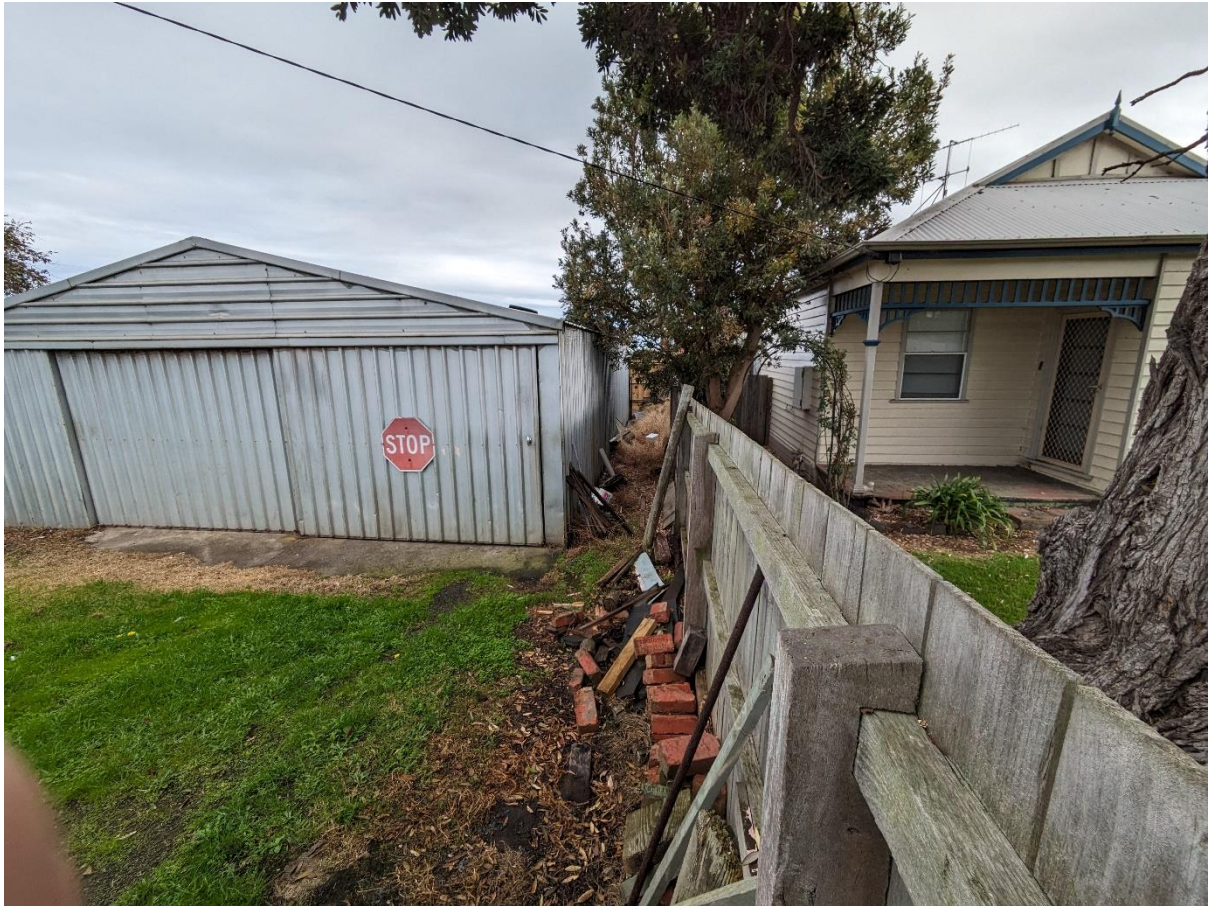
96 Bank St demolition
