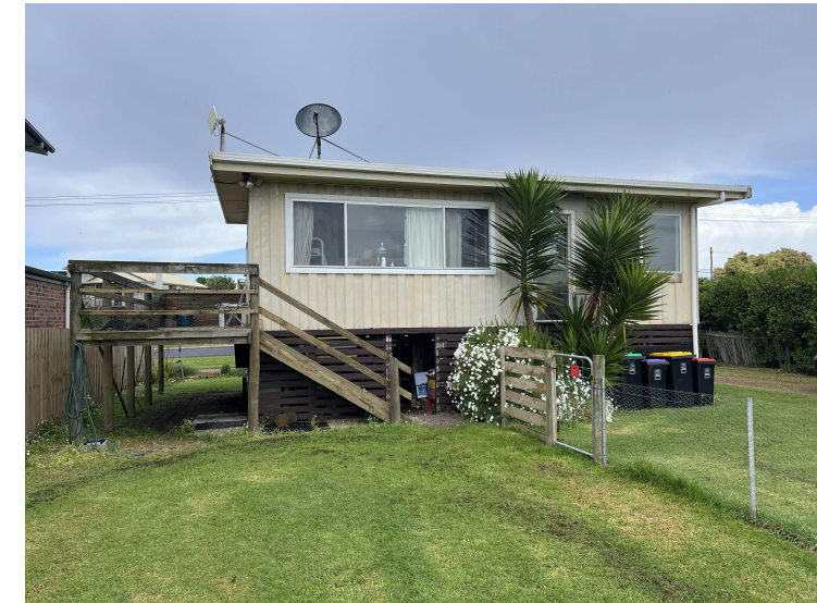
EXIST RESIDENCE: REAR NORTHERN VIEW
