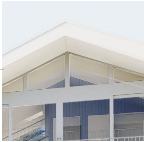
Fascia and Soffit lining, painted white
