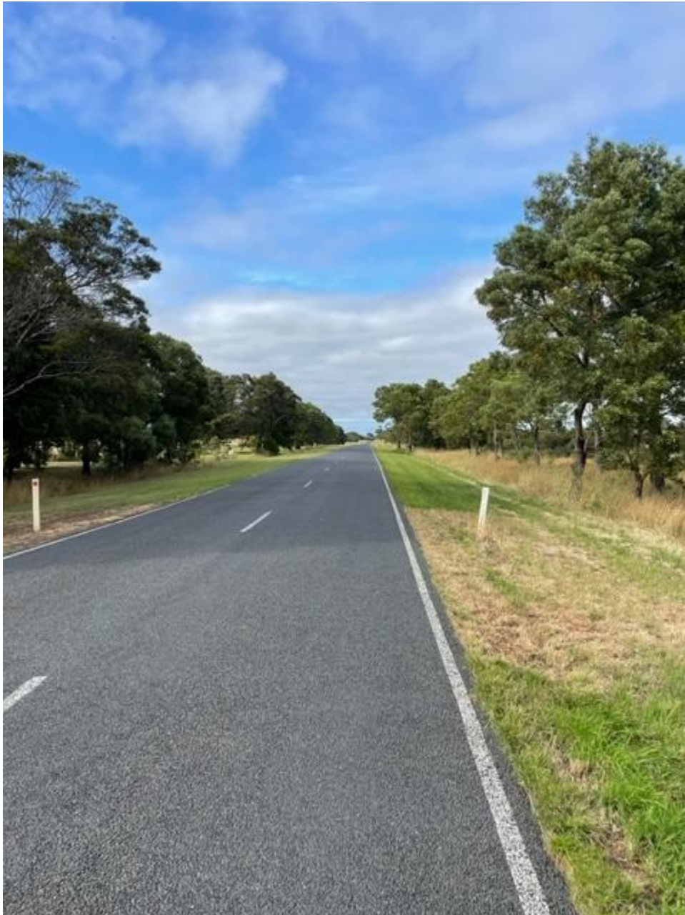
Photo 2 – View south along Koroit-Woolsthorpe Road from site access location
