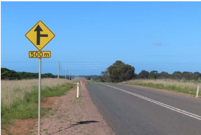
HEXHAM-WOORDOO ROAD FACING SOUTH APPROACHING ENTRANCE.
