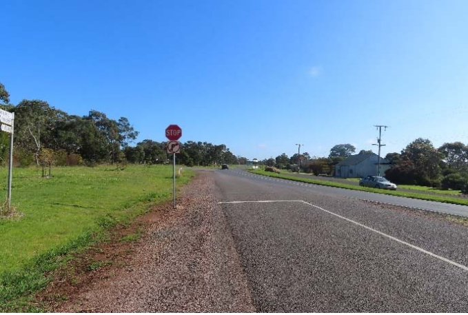
MORTLAKE-ARARAT ROAD & HEXHAM-WOORNDOO ROAD INTERSECTION FOR NORTH BOUND TRAFFIC FACING STOP SIGN.
