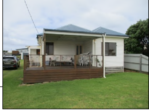
Existing Dwelling on No 35 Hamilton Street - Proposed Lot
