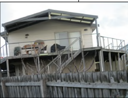
No 30 Robertson Street - Rear yard
