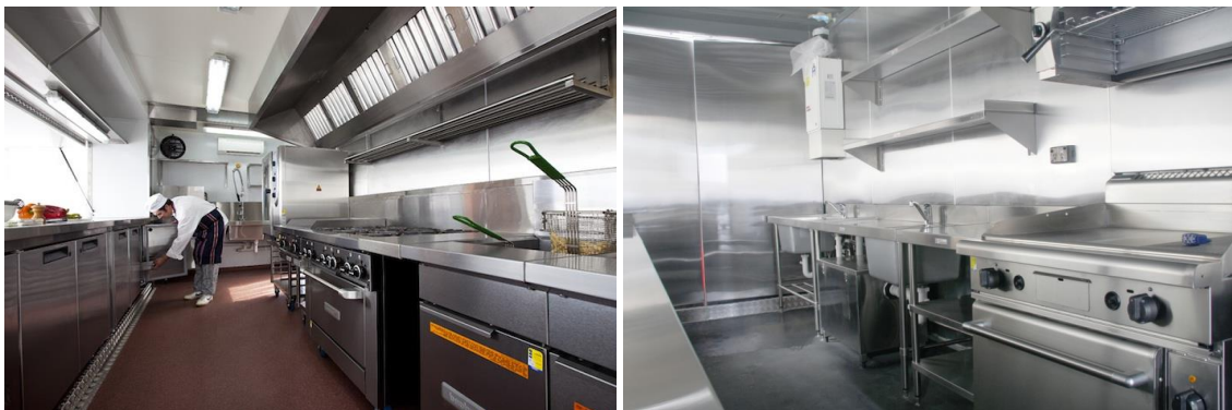
Figures 1 & 2 – Modern commercial kitchens dominated by stainless steel surfaces.
