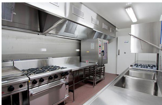
Figure 3 – Effectively planned kitchens enhance food safety risk management practices.
