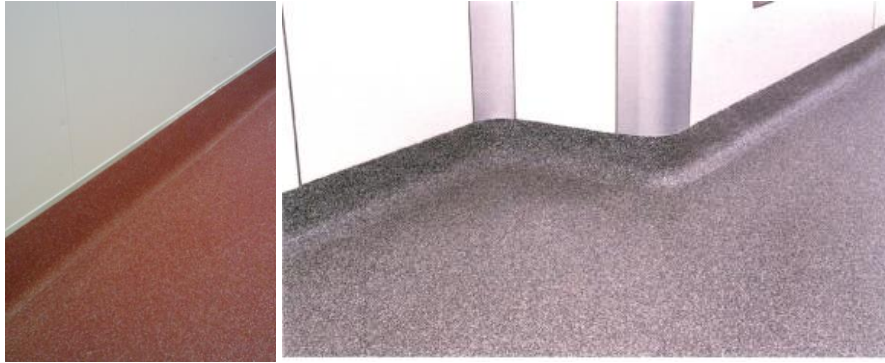
Figures 8 & 9 – Coving aids effective cleaning and reducing potential for pathogen accumulation.
