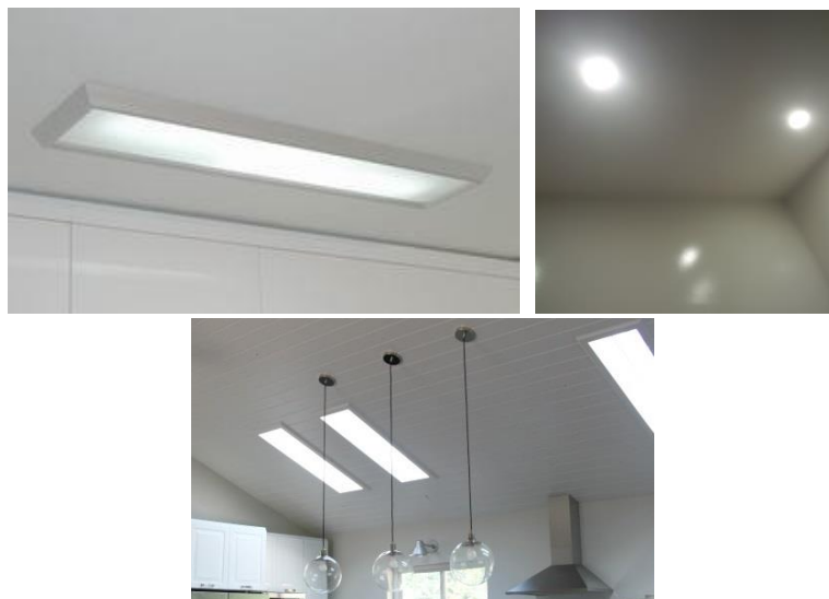
Figures 22-24 – For ease of cleaning, light fixtures should be recessed into the ceiling or fitted flush to the ceiling.
