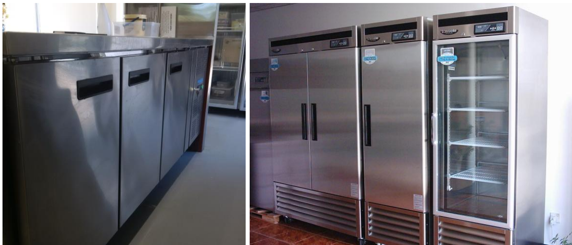
Figures 25-26 – Refrigerators and display cabinets must be able to keep food at or below 5degC; freezers must keep food frozen (<15degC).
