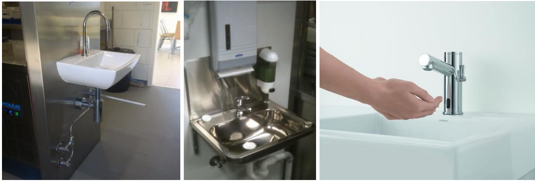
Figures 19-21 – Hand wash basins must be no further than 5 metres from any place where food handlers are handling food.
