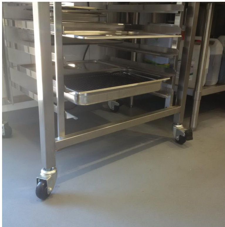
Figure 11 – Floors must be smooth, impervious, and free of cracks and crevices.
