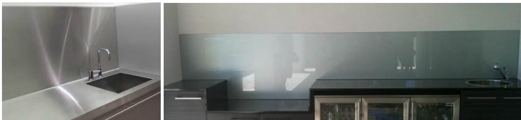
Figures 27-28 – Splashbacks should be carried to a height of 450mm above bench tops, hand wash basins, and similar fittings.
